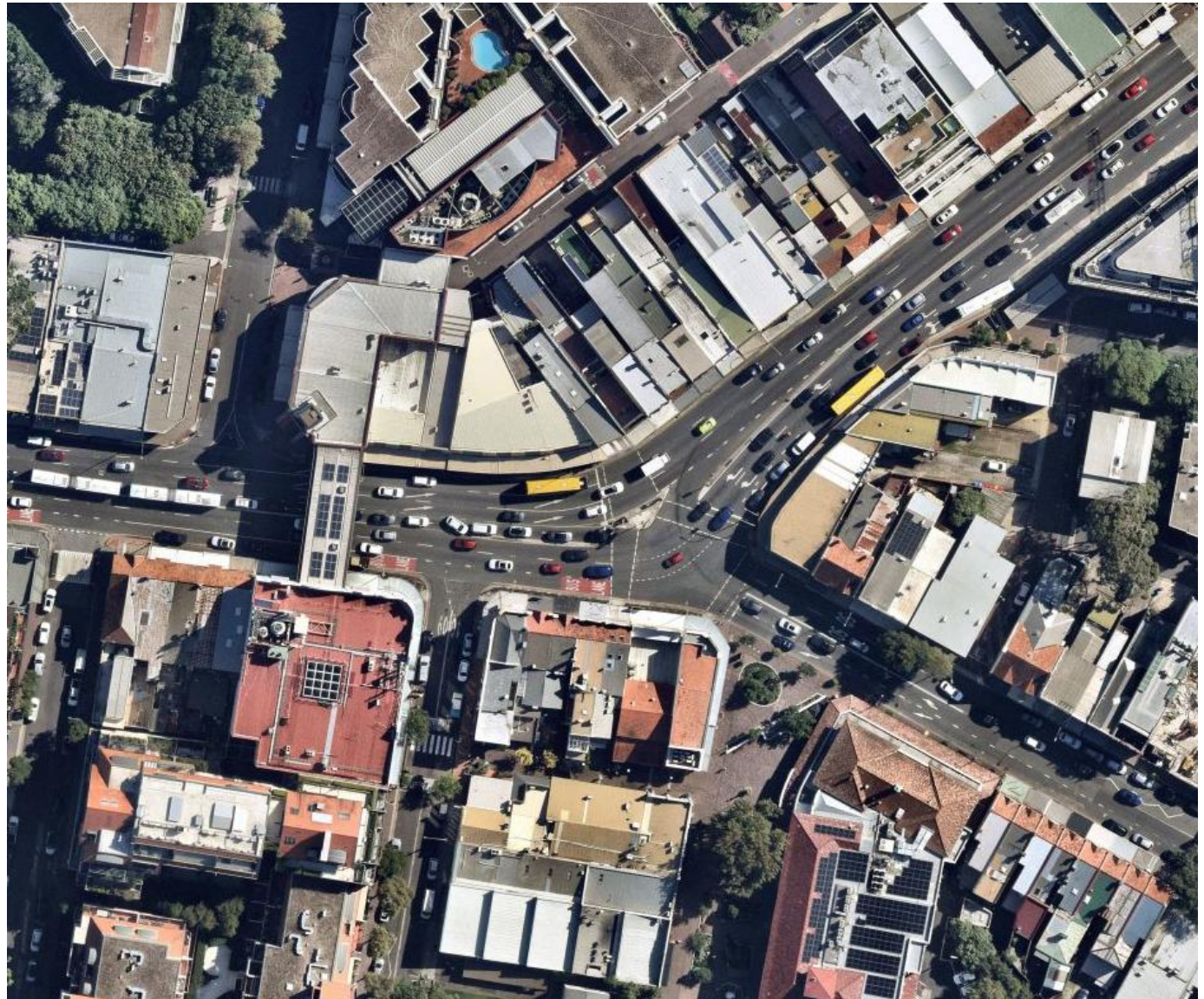
Figure 15: The Spit Junction, one of the key constraints in the road network
